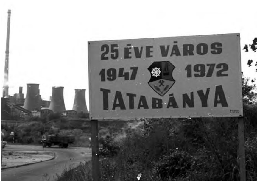
Power plant in Tatabánya, circa 1975
