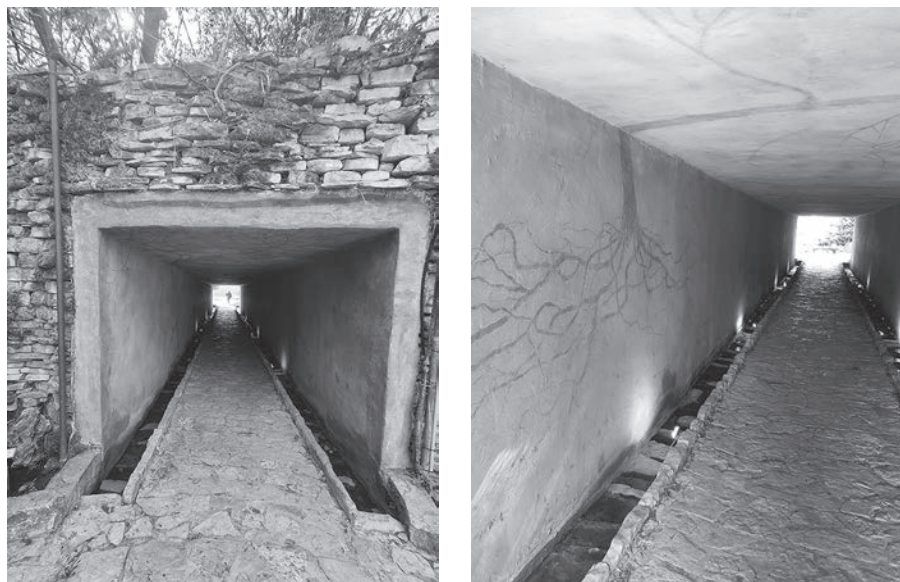
Fig. 17. Two views of the roots tunnel. (Photographs by the author.)
