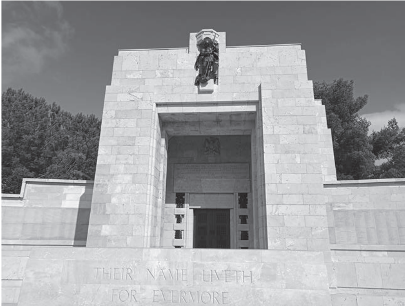
Fig. 8. The Stone of Remembrance and the Memorial Chapel. (Photograph by the author.)
